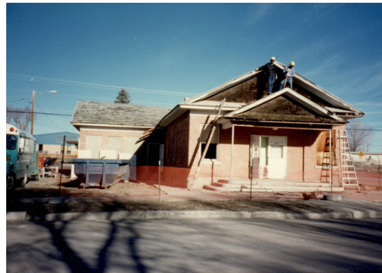
The Oddfellow/Rebekah Hall being torn down.
